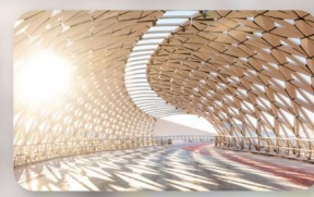
Ayrau Bridge Astana
